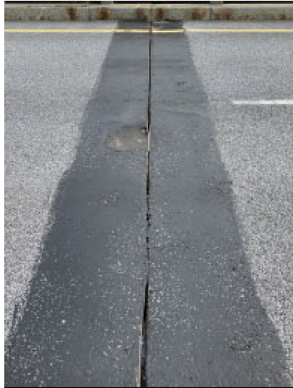
Vertical Steel Plate Joint & Asphaltic Plug over Pier #1 (left) and Pier 3 (right)
