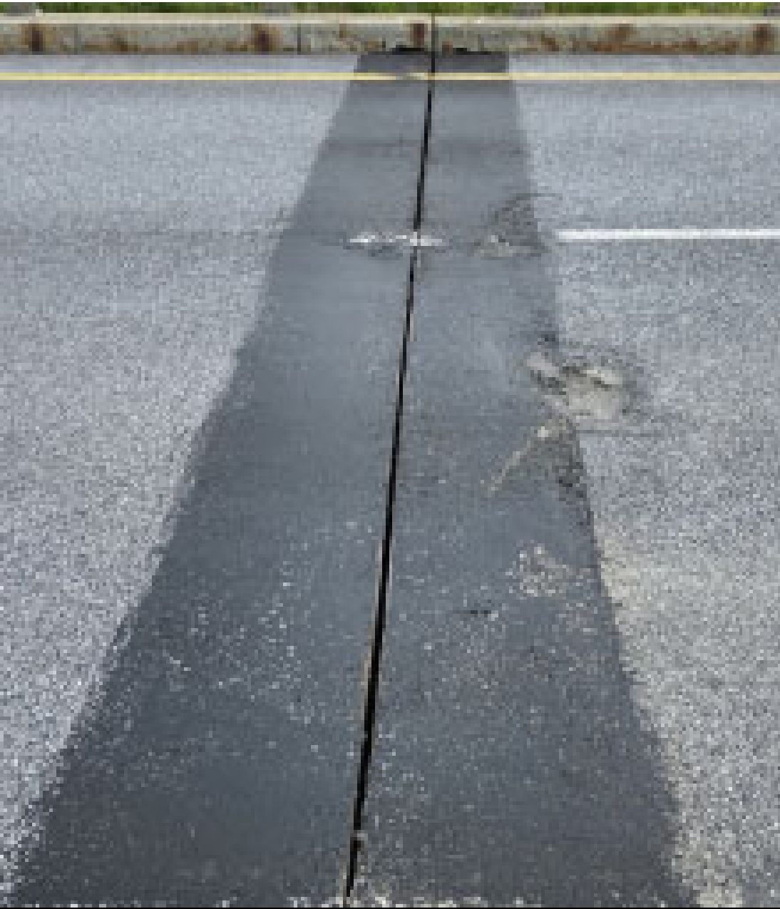
Vertical Steel Plate Joint & Asphaltic Plug over Pier #1 (left) and Pier 3 (right)
