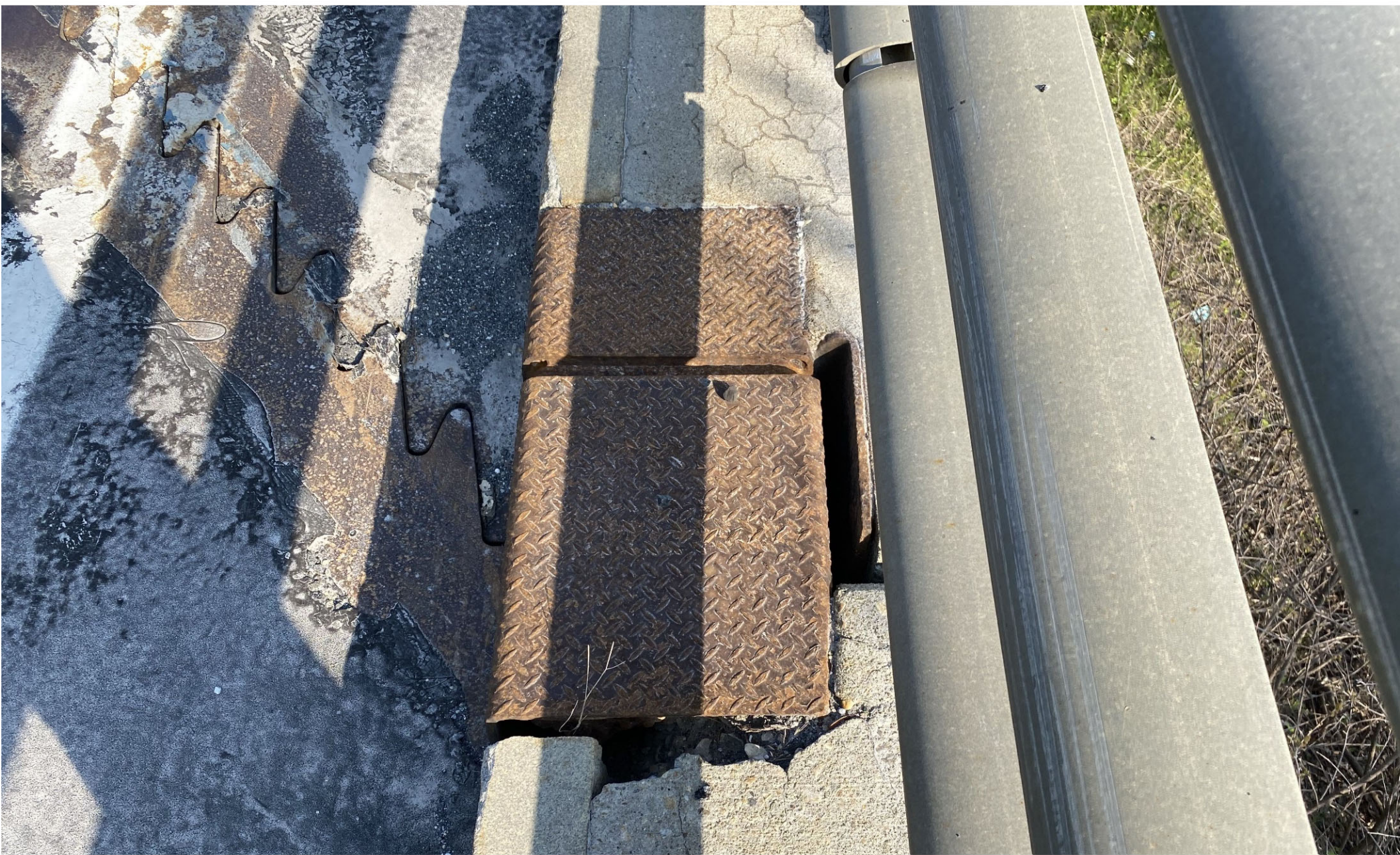
Concrete Spalling Surrounding Steel Joint at Abutment #2 on North Side
